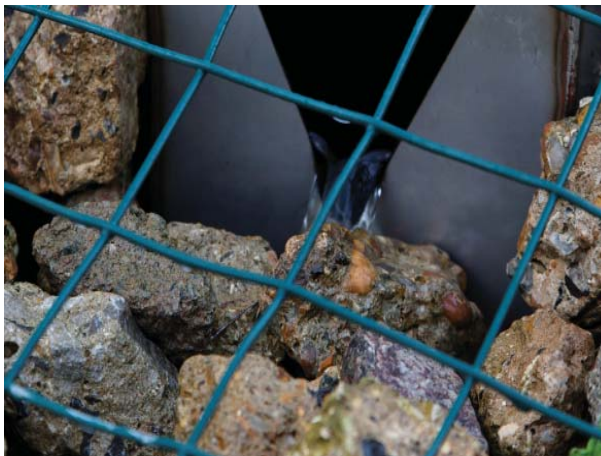
Recycled concrete used in a control structure in Cambourne, Cambridgeshire
