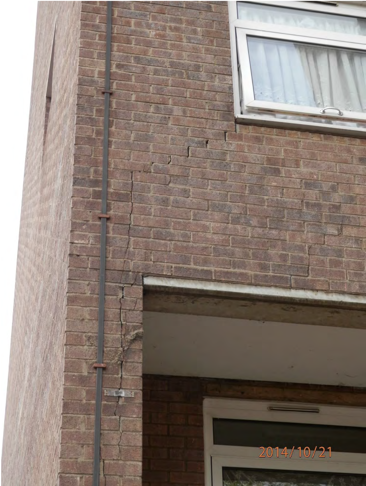
Year 1 and 2 Emergency Repairs due to wind loading acting with dead and live loading
