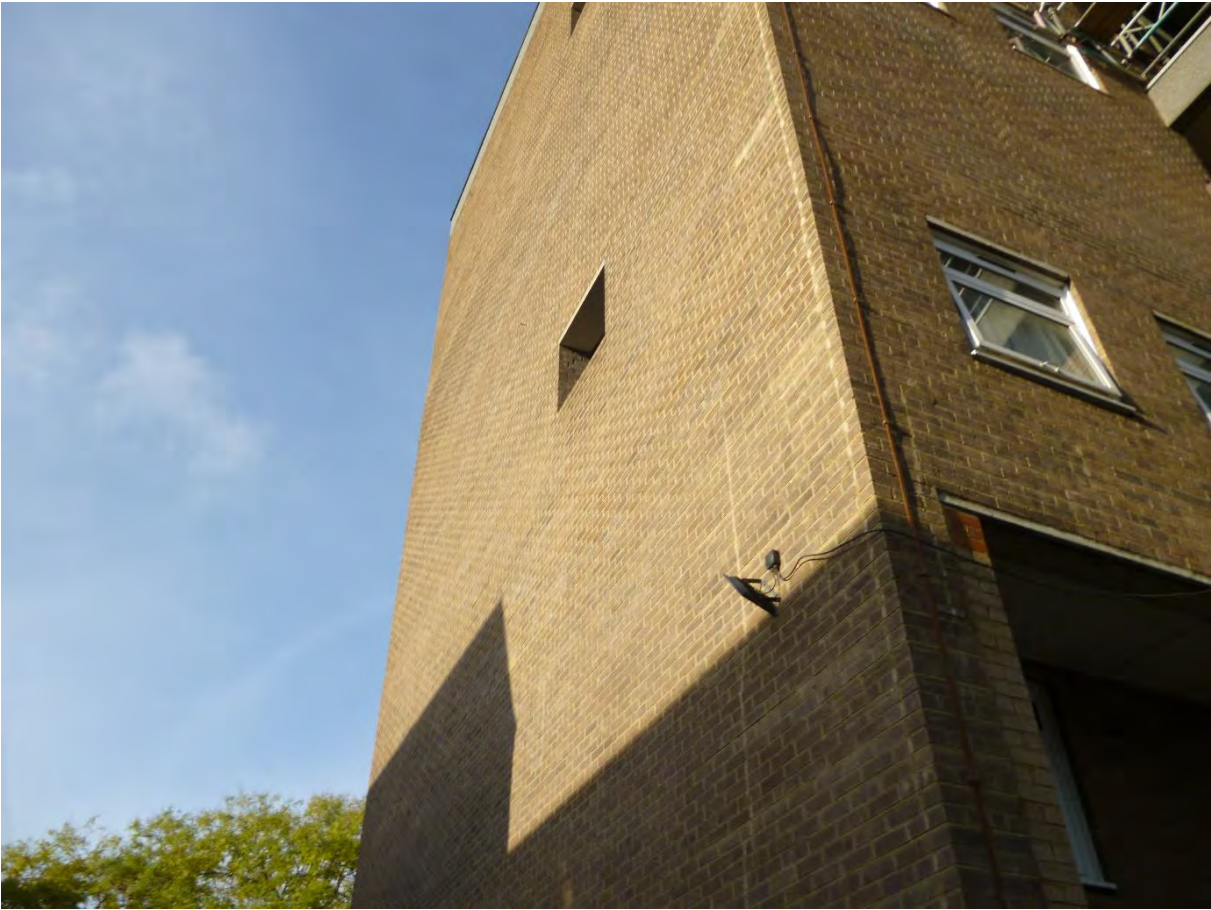
Corner of Hanover Court after Urgent Repairs 2017 / 2019 (Year 1 and 2)
