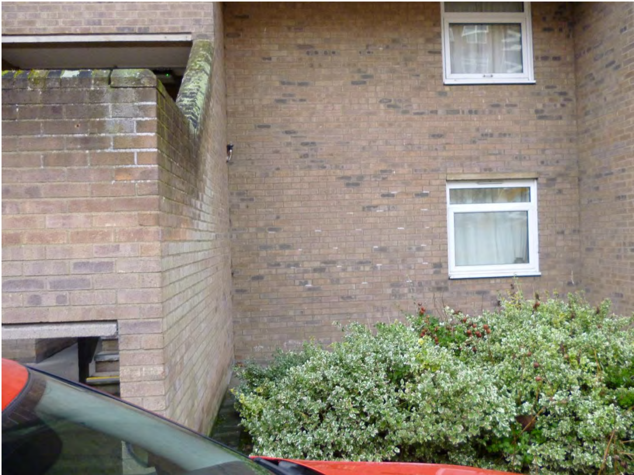
Princess Court Sample Panel – Tracing Brickwork Ties with metal detectors
