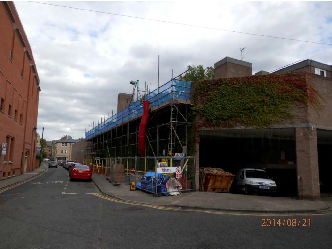
External View - Before the Year 0 Remedial works
