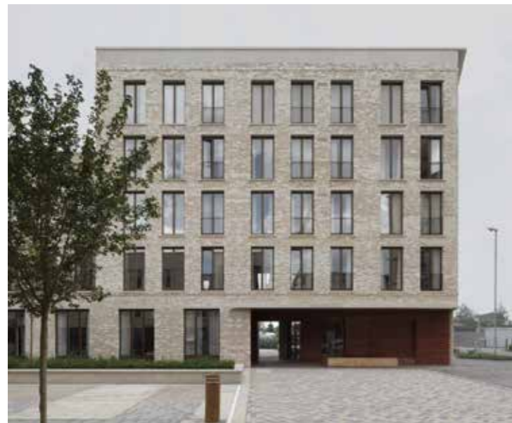
Material change to pick up communal entrances and amenity Wetherford Watson Mann, Ryle Yard
