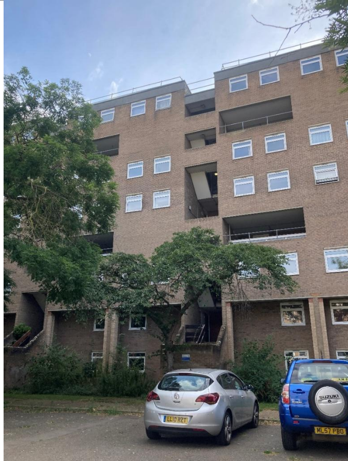
Plate 18 - View of the Site from outside number 18 George IV Street.
