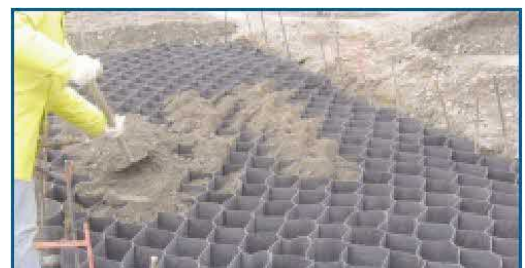
Figure 4. Static loading tests of up to 300kN/m2 revealed only minimal deflection (<5mm) of the surface of filled Geocell
