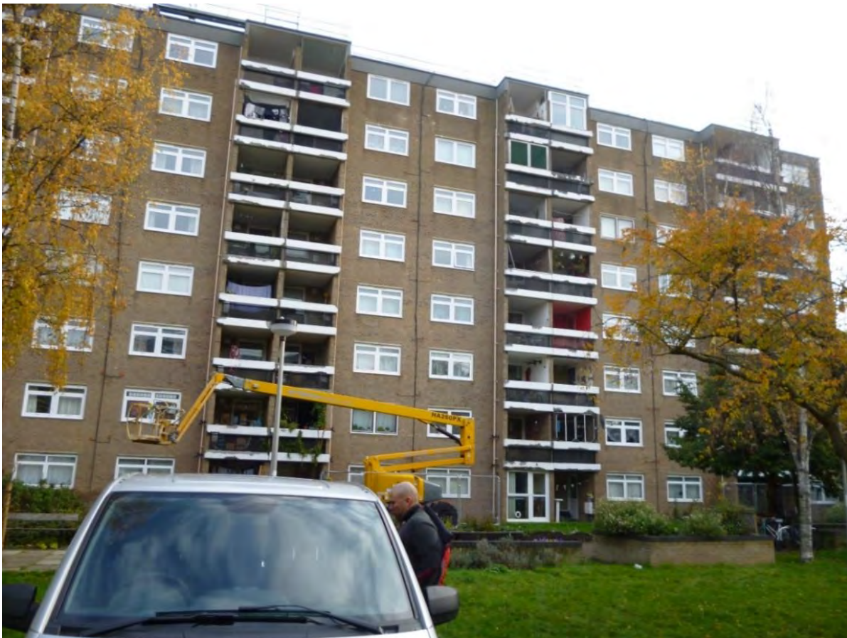
Hanover Western Side - Note the mobile access platform used to access and repair Hanover Court Building initially the Parapet panel Repairs and then the Balcony panels Tap Testing to remove loose concrete. .
