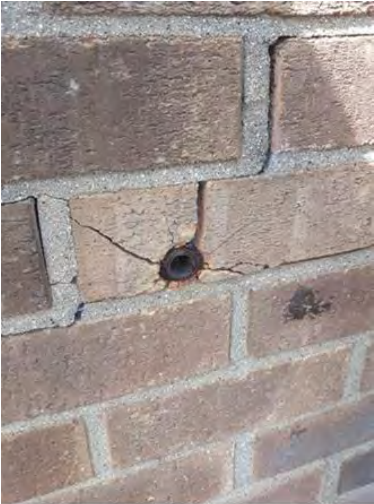
Top of Princess Court Bin Chute Tower corroded old Scaffold Fixing bursting the brickwork at High level
