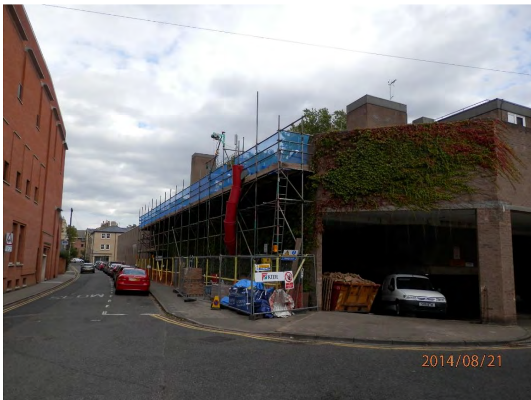
External View - Before the Year 0 Remedial works
