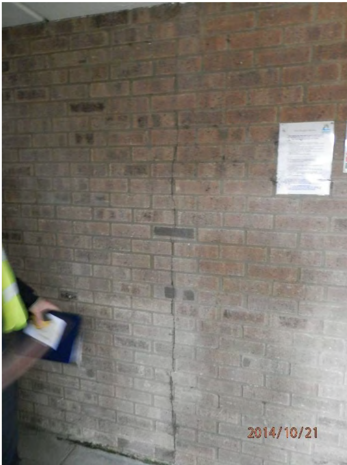
Eastern Staircase of Hanover Court Typical Entrance Structure - Cracking Internal Northern Side: Repaired in Year 1 Urgent Works
