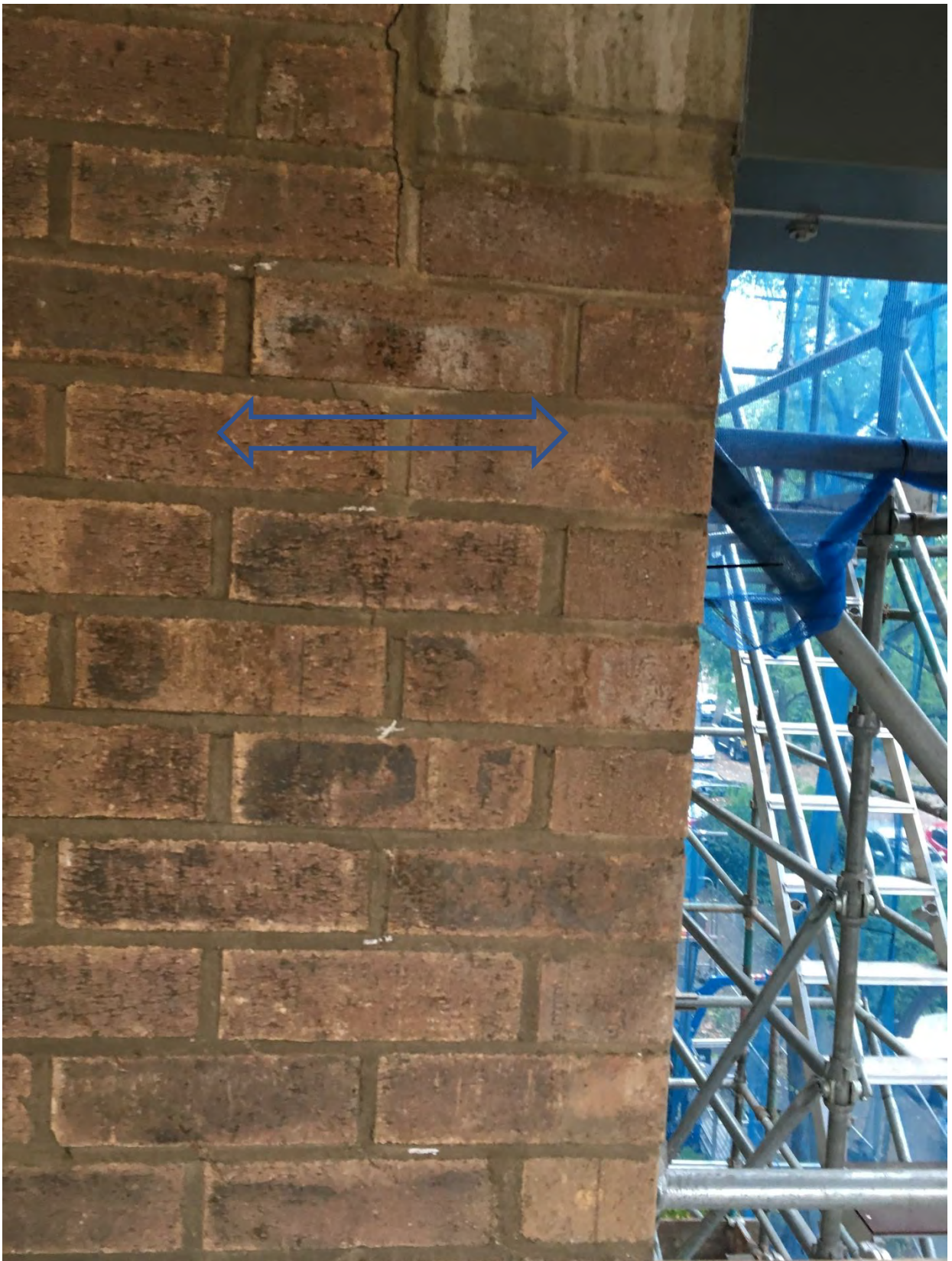
Cracked Walkway Beam Bearing onto the Hanover Court Building – Note the tracing of the brickwork ties
