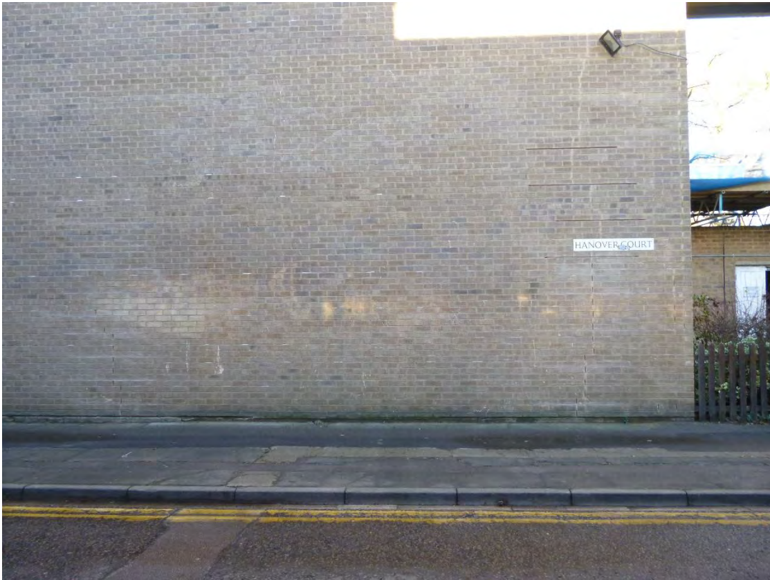
Hanover Court Sample Gable End Panel Tracing Brickwork Ties – Note the unusual pattern
