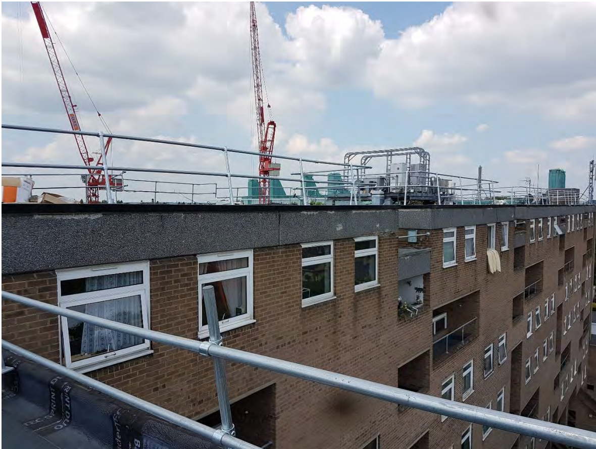
General View of North Eastern Elevation Typical Parapet Panel Tap Test in Year 1 Prior to Year 2 Sika Repairs Sika 903 Sika 610 Sika 612 and Anti-carbonation Coating Sika 675
