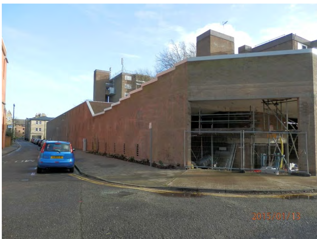
External View - after the Year 0 Remedial works and the reduced and tied back external wall located aside the car access ramp.
