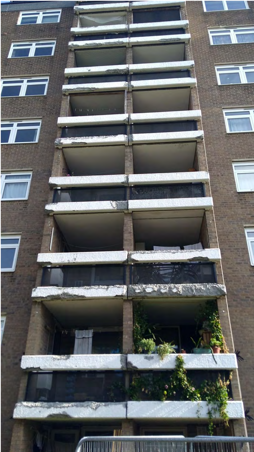
Hanover Court Tap Tested and Primed Panels with SIKA 903 and SIKA 610 Locally – Typical Example
