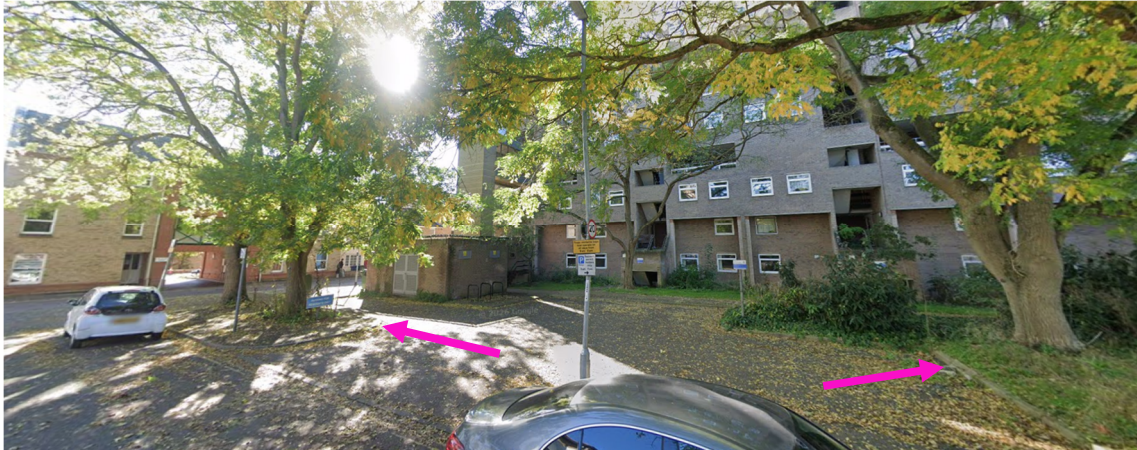
Image 2 – The existing car park to be used for the Demolition access. G002 is on the left side of the image and T003 is on the right side of the image. Temporary protective fencing to be installed at the kerb edges.
