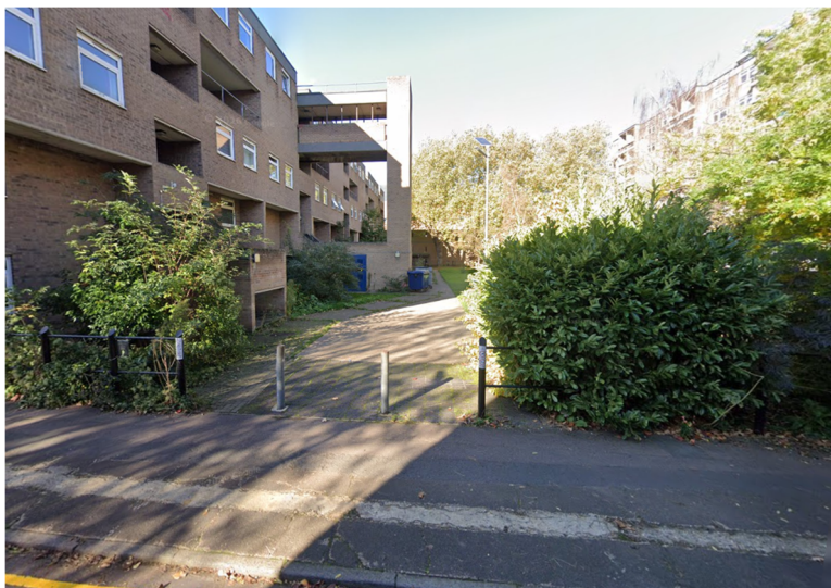
Image 3 – The demolition phase point of access off Coronation Street.
