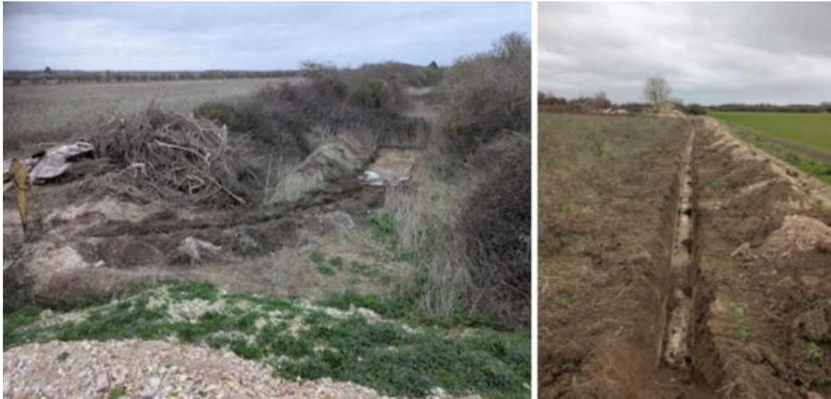
Installing the trench to the infiltration area. (EW, 2026)
