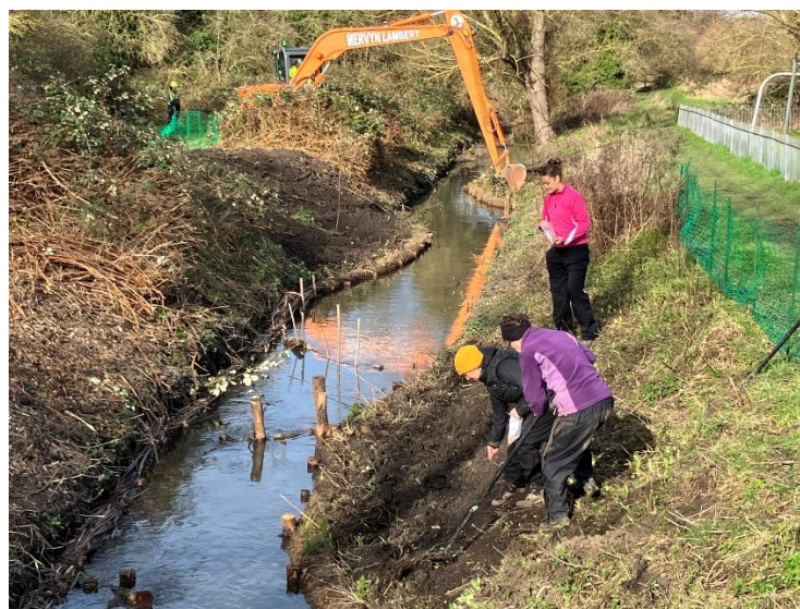
Volunteers and contractors Aquamaintain working along East Cambridge Main Drain.
