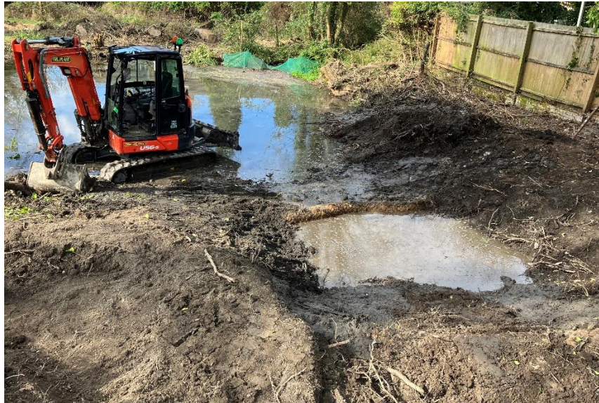
Aquamaintain installing pollution mitigation system at Giant's Grave
