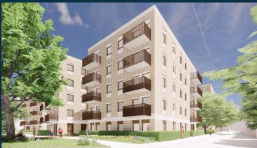
VIEW FROM THE CORNER OF CORONATION AND BENTINCK STREET
