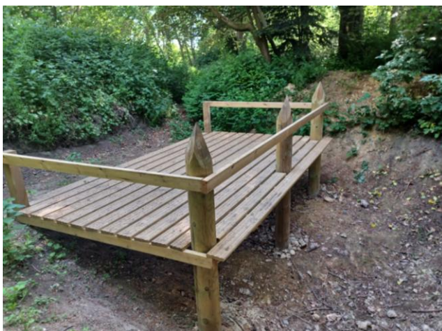
First dipping platform being installed at Patchwork Education Village
