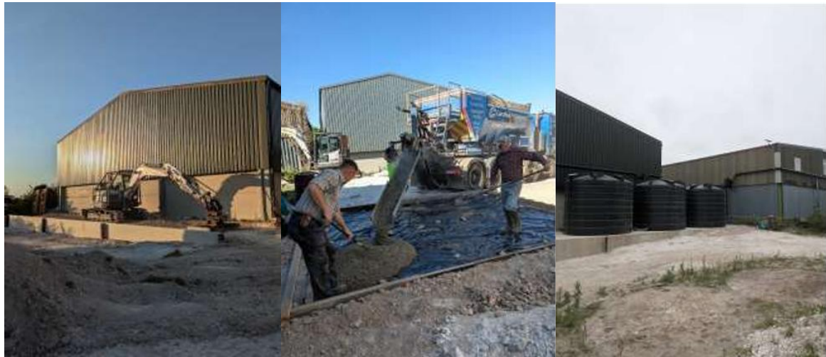
Rainwater Harvesting system being built at New Shardelowes Farm
