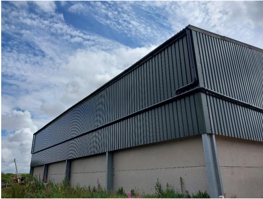
JRH Ltd installed roof rainwater capture pipe system
