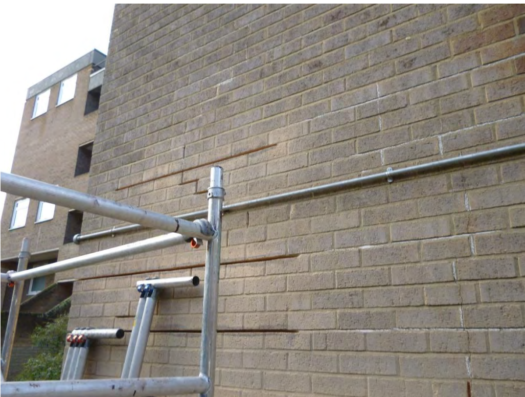
Example Repairs on Princess Tower
