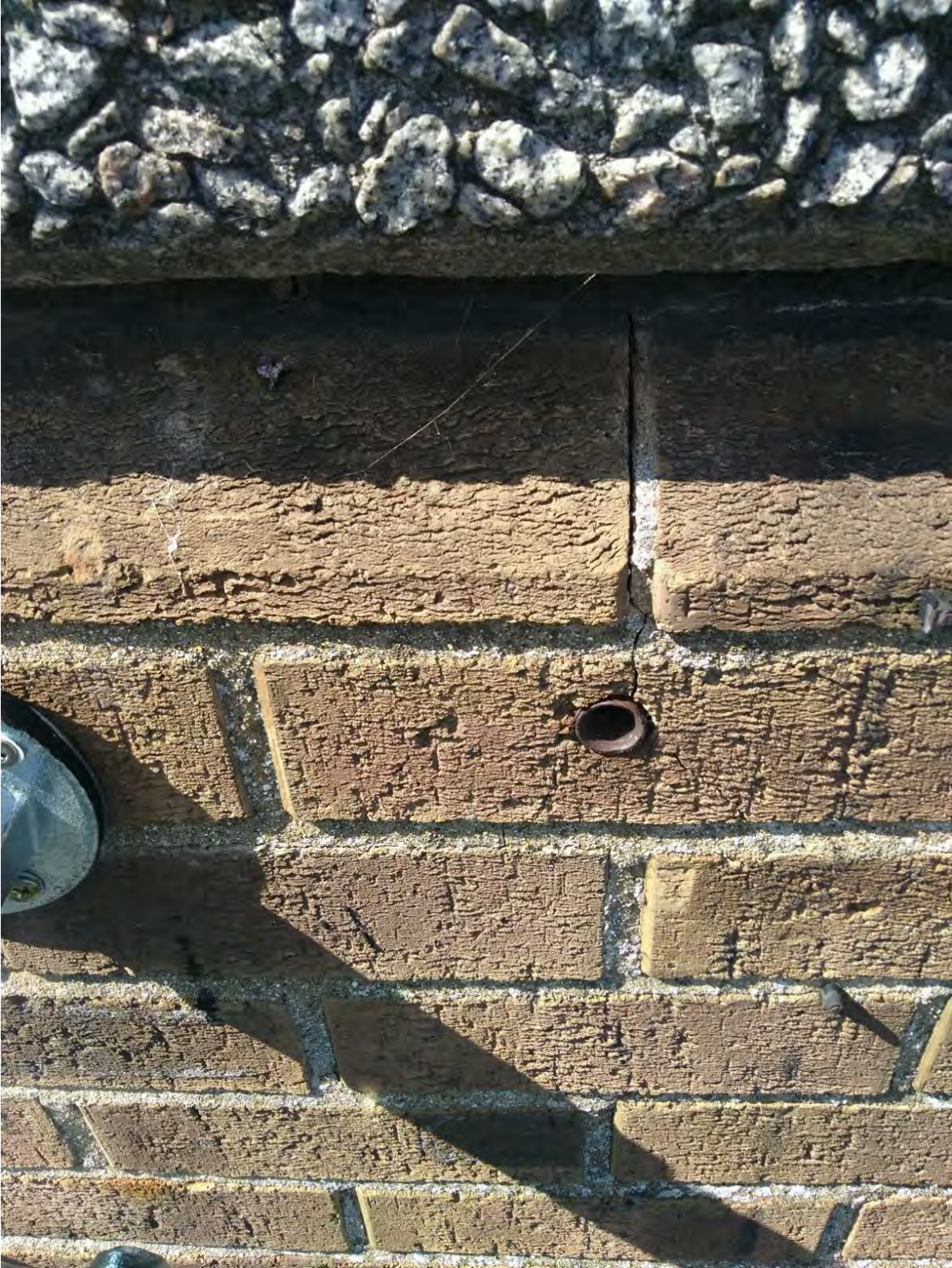
Typical Examples of Old Fixings left Rusting and Expanding within the Masonry Façade of the Buildings
