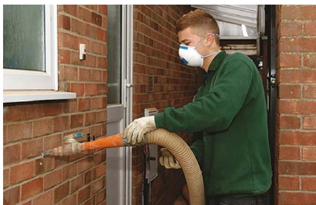
Fitting cavity wall insulation (© Aran Services)
