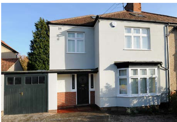
Retrofitted external wall insulation
