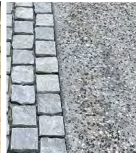
Material change from paver to gravel
