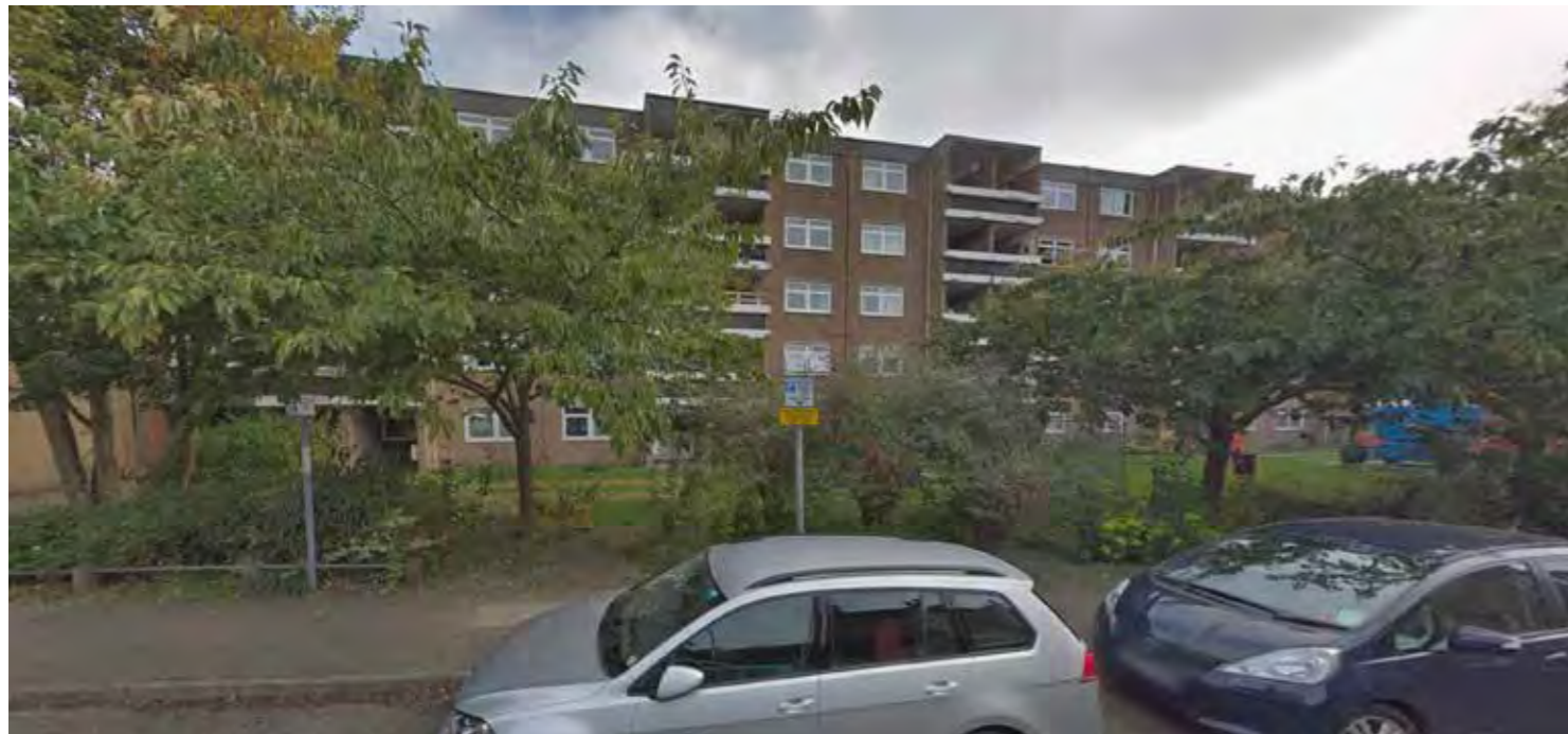
Existing Bentinck St
