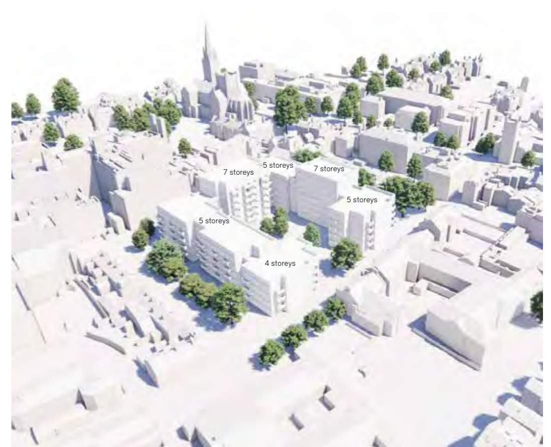
View from south west
