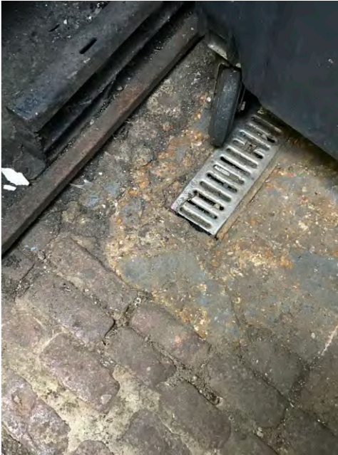
Photo showing existing fat drain
