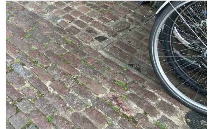
Existing recessed cover within setts
