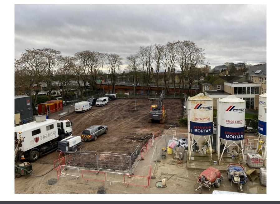
Following Demolition the site was remediated where required with contaminated material removed for treatment and disposal, All of these works where monitored and validated by our environmental specialists.
