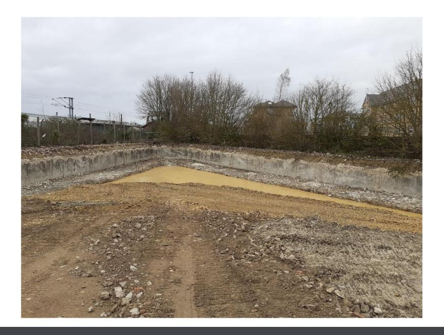
Following Demolition the site was remediated where required with contaminated material removed for treatment and disposal. All of these works where monitored and validated by environmental specialists.
