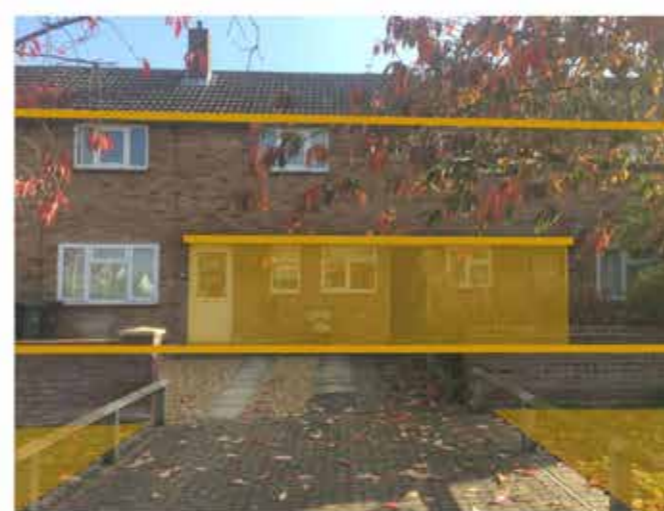
3. Two storey terraced houses with front gardens facing towards the high street - emphasis on entrance.
