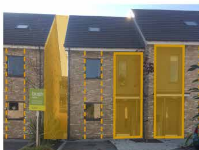
5. Two storey semi-detached houses with different materials used to emphasise vertical building elements. Accommodation situated within attic space.
