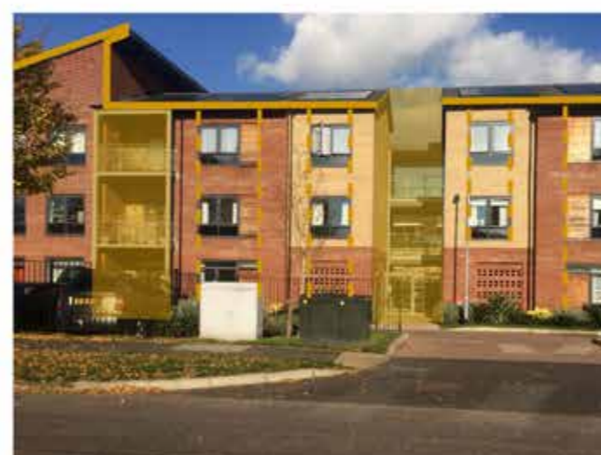
6. Three storey residential flat block with pitched roofs, projecting balconies and colour variations in the brickwork used to emphasise vertical building elements.
