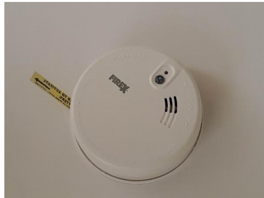
Heat detector located In the kitchen / diner
