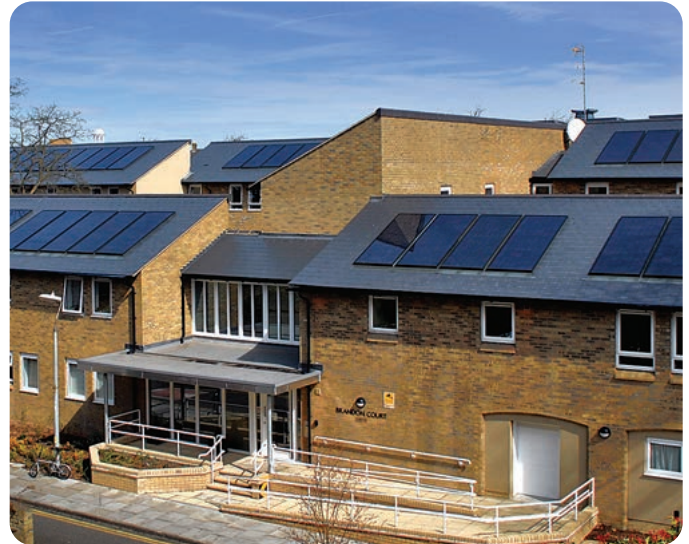
Solar photovoltaic (PV) panels at Brandon Court © Viridian Solar
