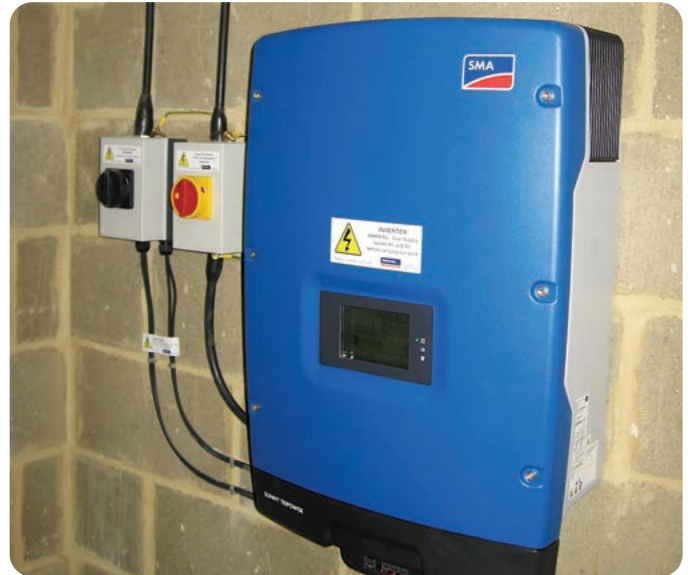
Inverter for solar photovoltaic system at Cherry Hinton Village Centre
