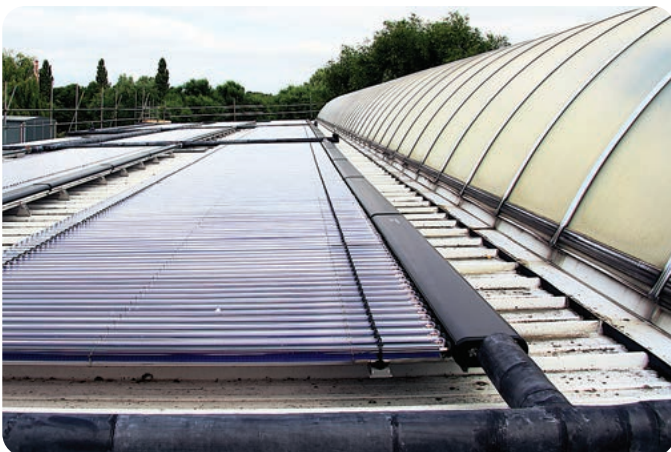
Solar thermal hot water system at Abbey Pool
