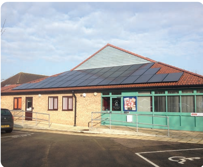
Solar photovoltaic (PV) panels at Buchan Street Neighbourhood Centre
