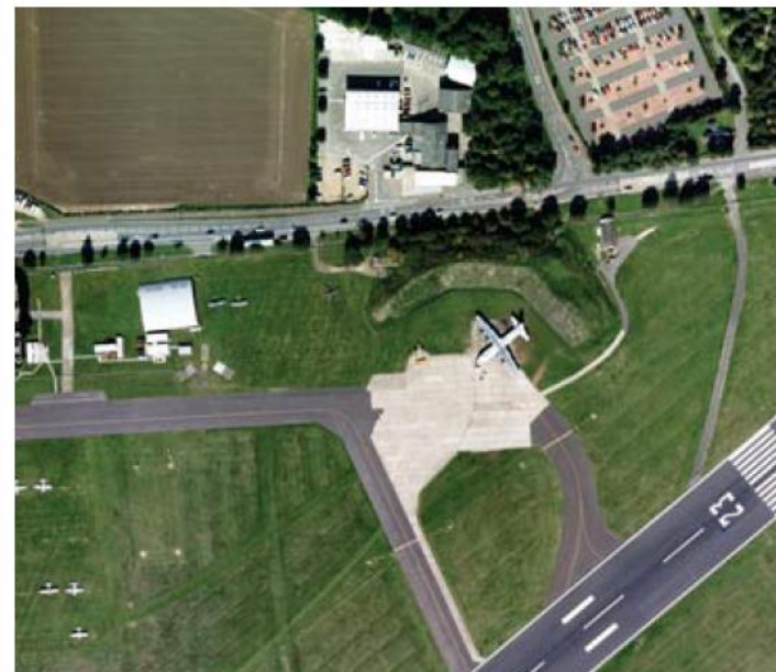
Existing engine run-up bay
