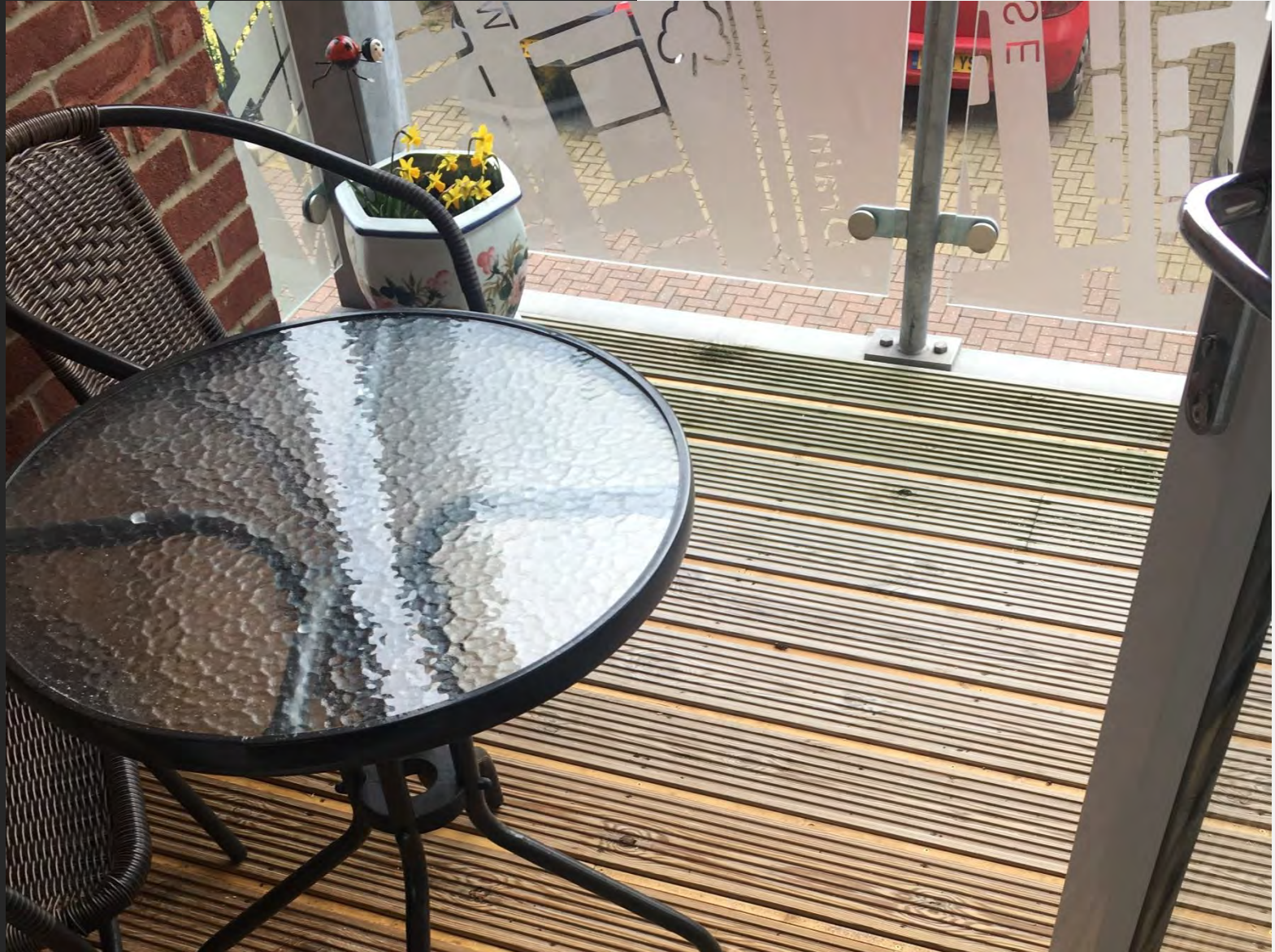
EIS: Balcony infills
