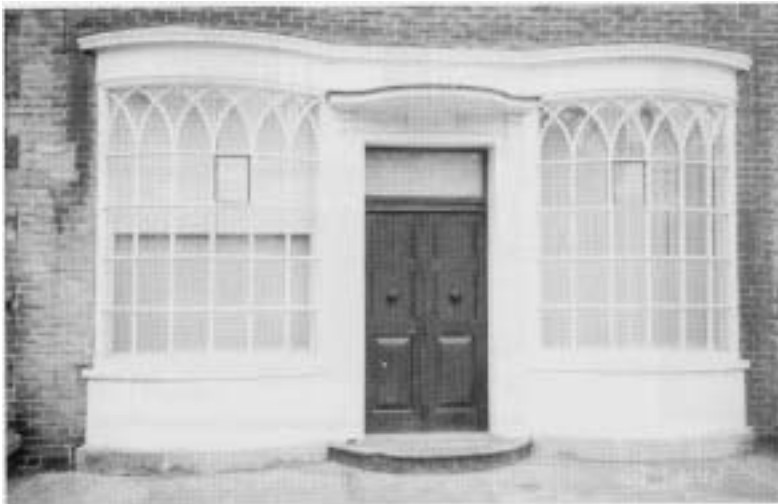
White painted bowed shopfront, Trumpington Street
