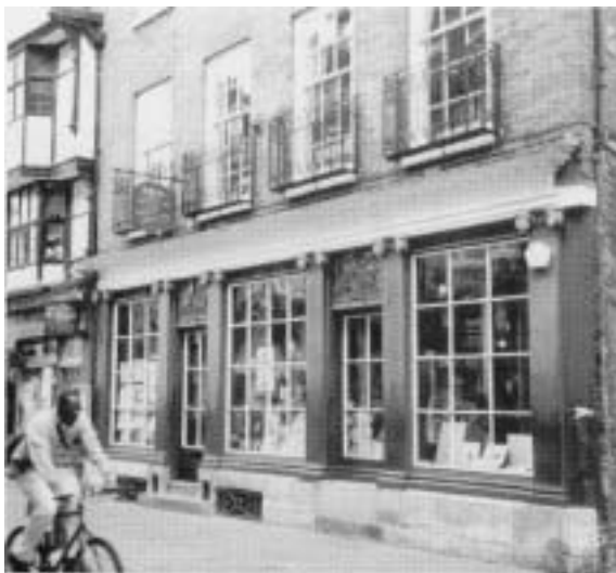
CONTRAST BETWEEN SHOPFRONTS OF THE EARLY AND LATE NINETEENTH CENTURY
