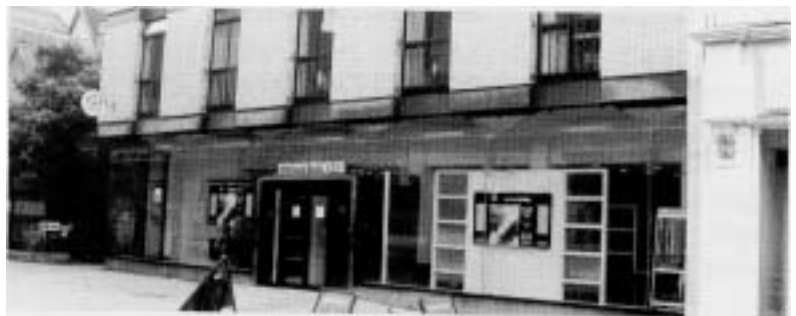
Modern light-weight shopfront, Peas Hill
