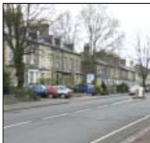
Poor frontages to terraces along eastern side of Hills Road
