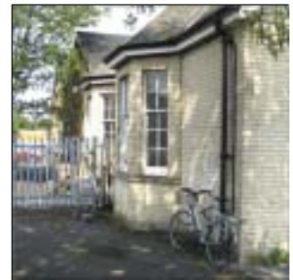
1932 Northern workshop/office building
