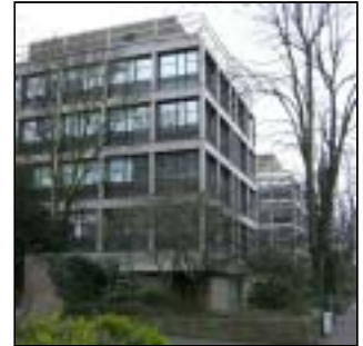
Office development along Station Road
