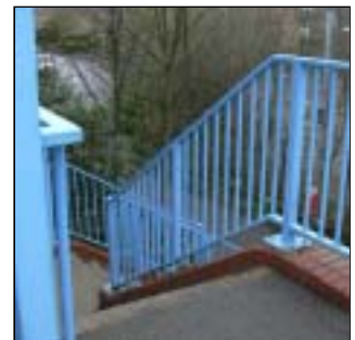
Existing pedestrian link on to the Carter Bridge
