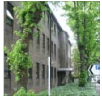
Daedalus House, Station Road
