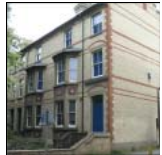
Wilton Terrace, 32-38 Station Road
