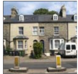
Eastbourne Terrace, 89-91 Hills Road
