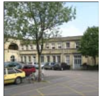
Cambridge Station – southern wing
