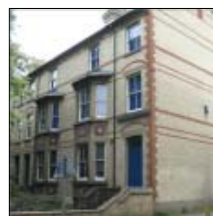
Wilton Terrace, 32-38 Station Road
