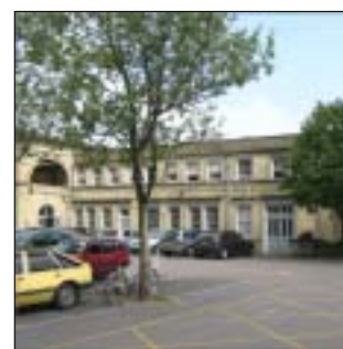
Cambridge Station – southern wing
