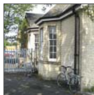
1932 Northern workshop/office building
