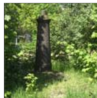
Crane Base on the 'Triangle Site'
