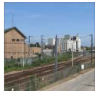
Panorama across to mill from Hills Road bridge
