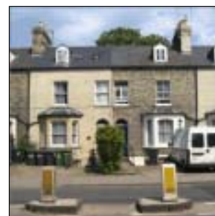
Eastbourne Terrace, 89-91 Hills Road
