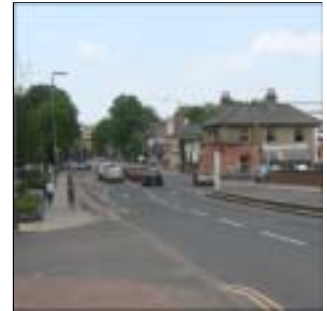
View along Hills Road from railway bridge looking north
