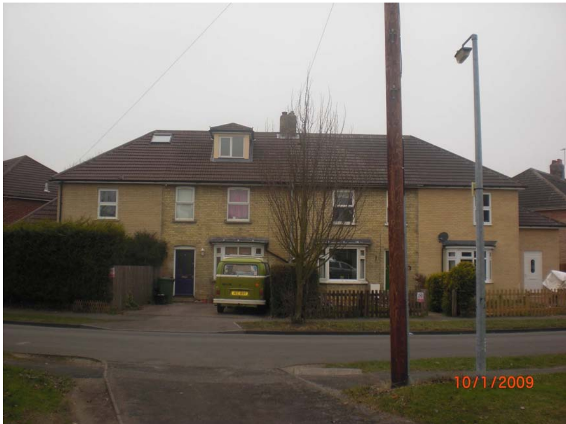
CIMG0241 Row of 4 terraced houses
