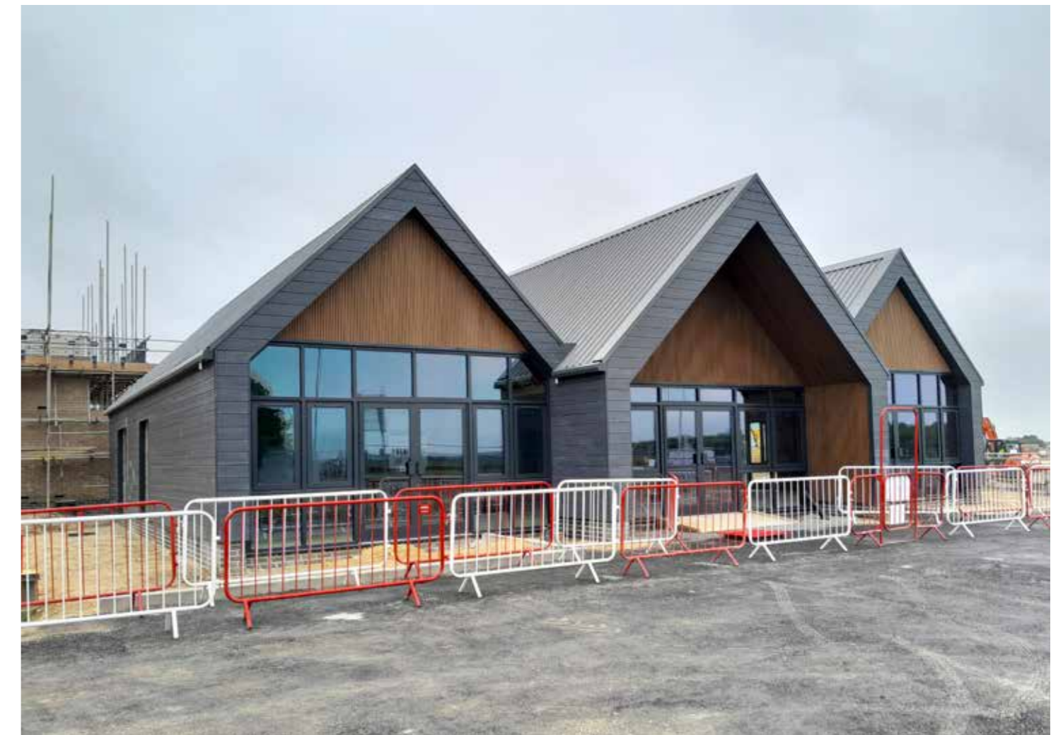
Sales & Marketing Temporary pavilion building under construction
