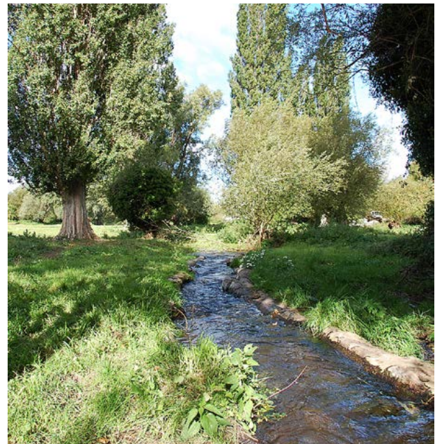
The Rush, a natural bypass channel to aid fish passage at Sheep's Green
