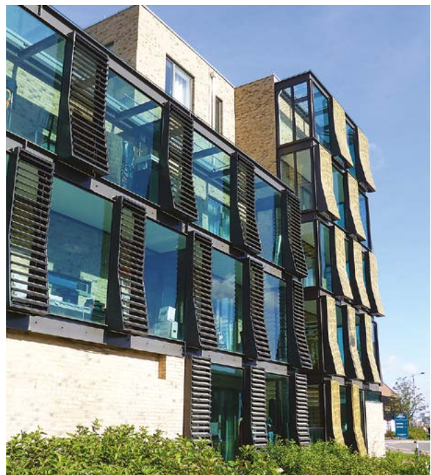
Apartments with ‘Winter Gardens’ at Clay Farm
