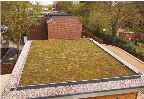
A green roof helps slow down rainwater run-off
