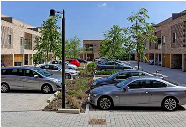
Permeable paving at Abode on Clay Farm
