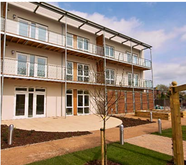
'Brise soleil' help to control solar warming
