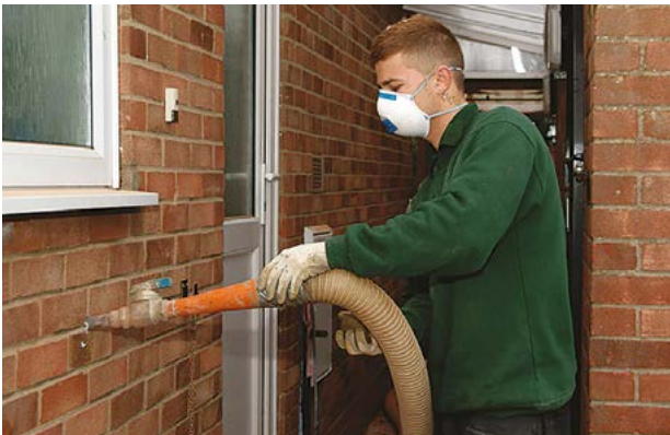
Fitting cavity wall insulation (© Aran Services)
