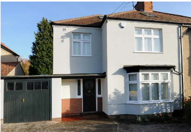
Retrofitted external wall insulation
